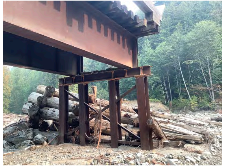
Right Bank Abutment when facing downstream
