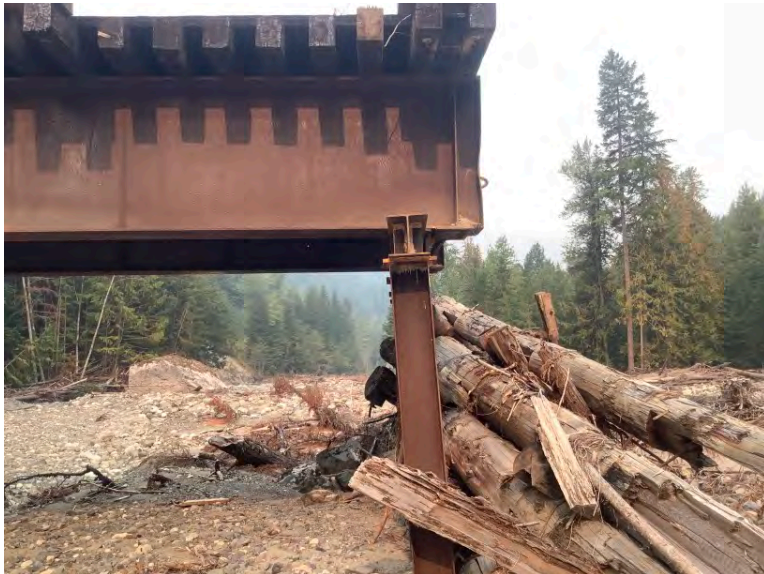
Right Bank Abutment when facing downstream
