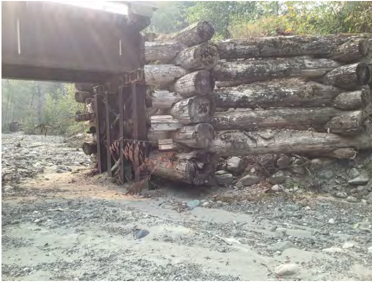
Left Bank Abutment when facing downstream
