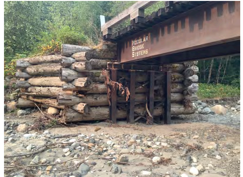
Left Bank Abutment when facing downstream
